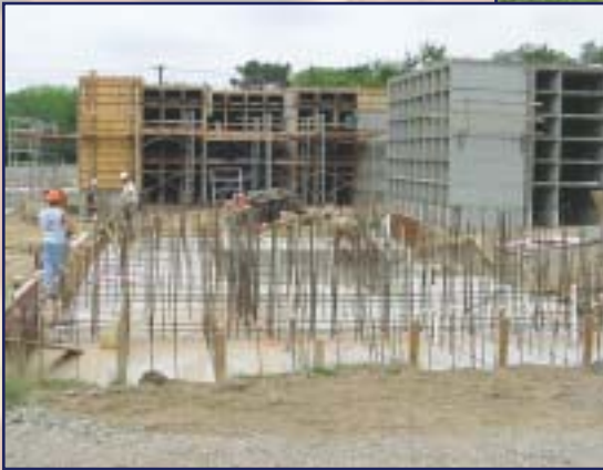
Garden Conservatory Mausoleum construction
