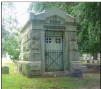
Swan Callendar Mausoleum, Evergreen Plot - While the Fitch Memorial was under construction, the playwright's remains were kept in the tomb of a friend.
